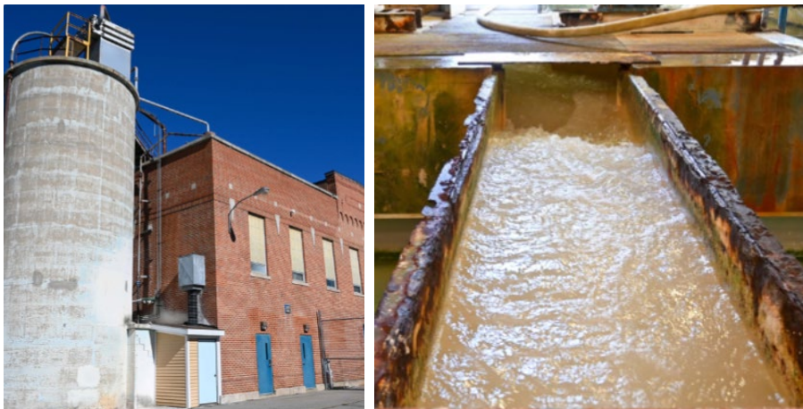
City of Batavia Water Treatment Plant
