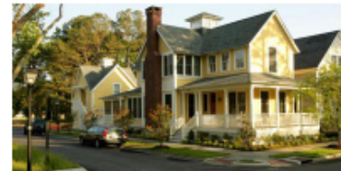
3.3 A successful corner lot creates a strong frontage along both the primary and secondary streets. Landscaping elements soften the hard edges of the building along the front and side setbacks.
