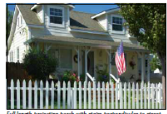
Full-length projecting porch with stairs perpendicular to street.
