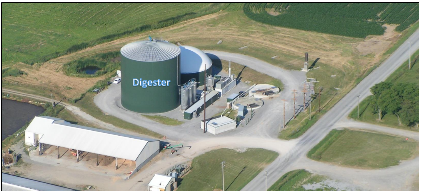
Photo #2: Digester Sky View
