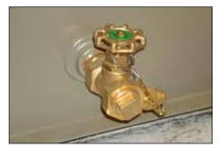
Figure 3. Drain valve with sampler.
