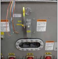
Figure 8. VFI transformer with visible break.
