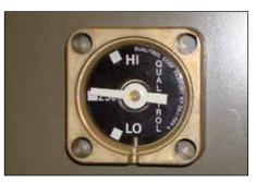
Figure 5. Liquid level gauge.
