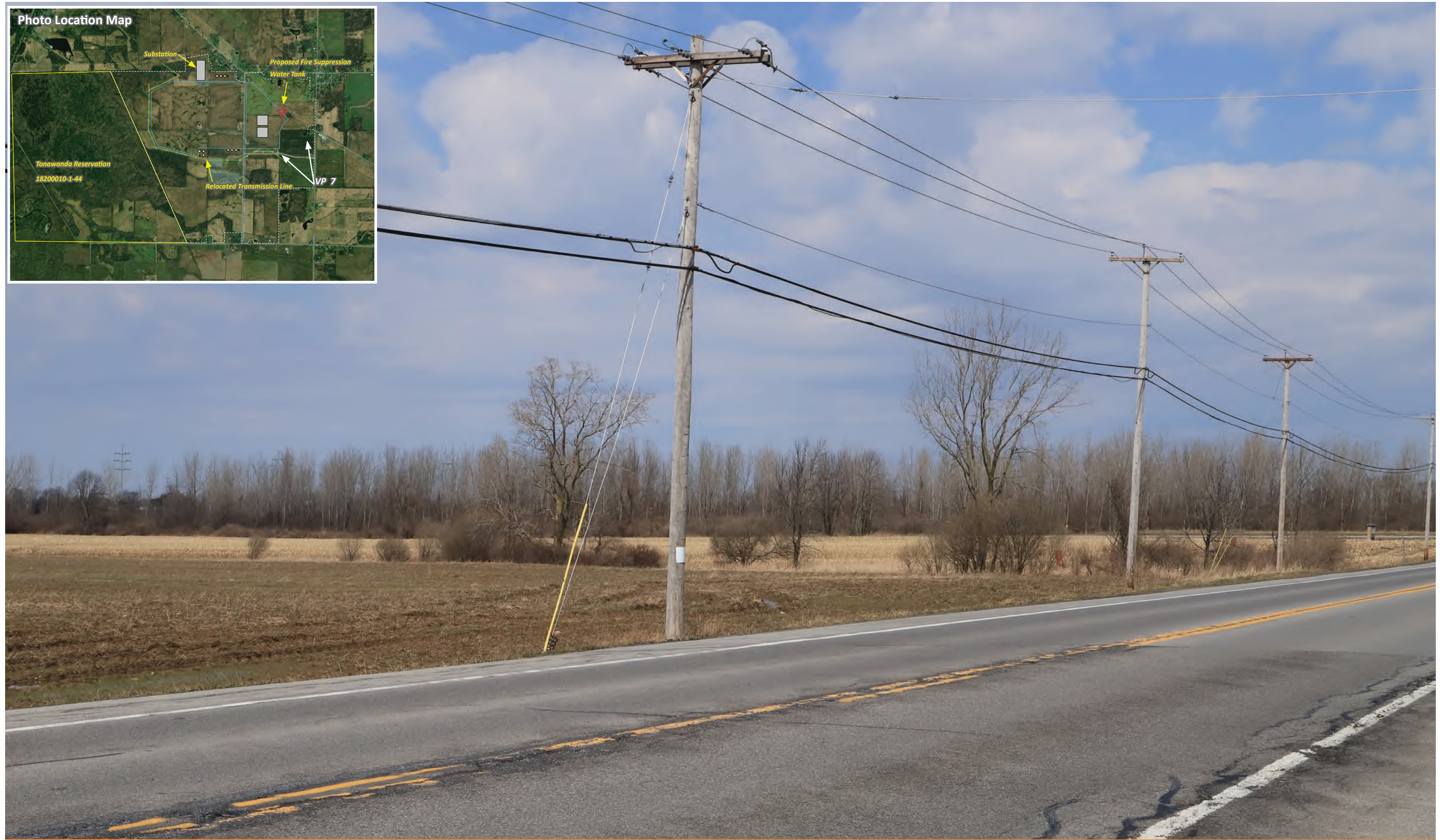
PHOTO 7 ALLEGHENY ROAD EXISTING CONDITION
