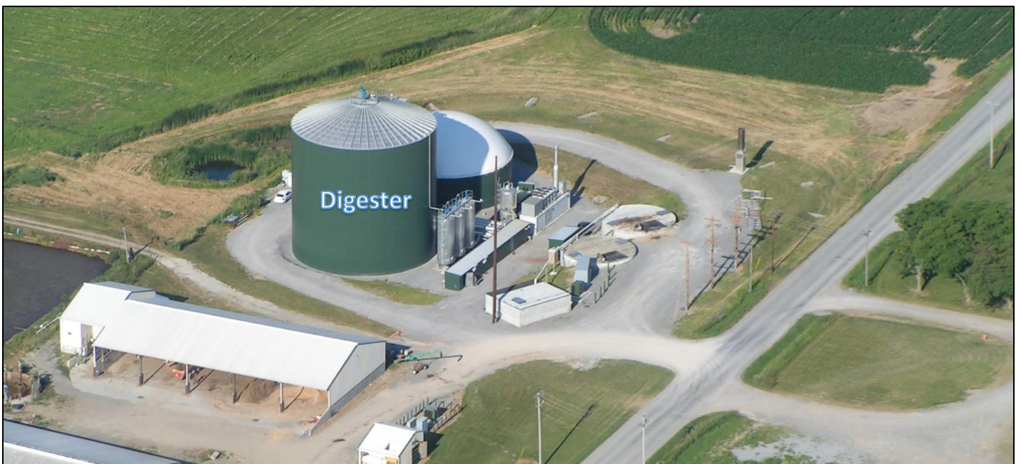
Photo #2: Digester Sky View
