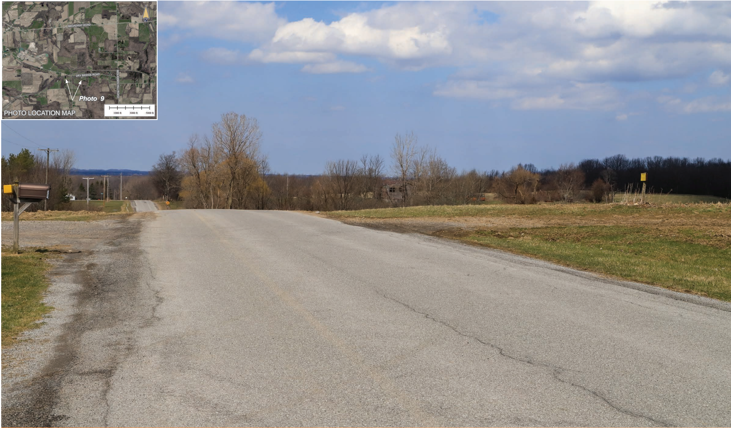
Photo 9 - Chaddock Rd near # 11080 EXISTING CONDITION
