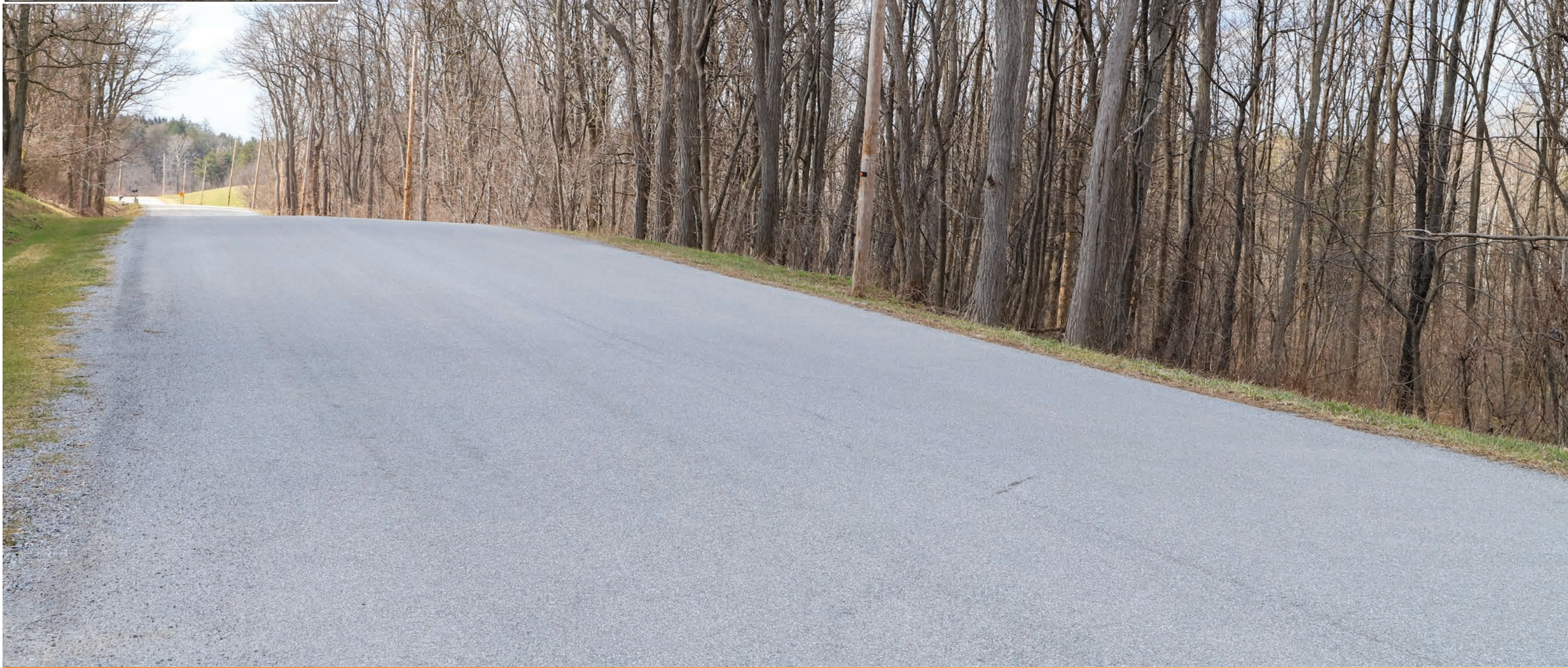
Photo 5 - Dry Bridge Rd near # 4338 EXISTING CONDITION
