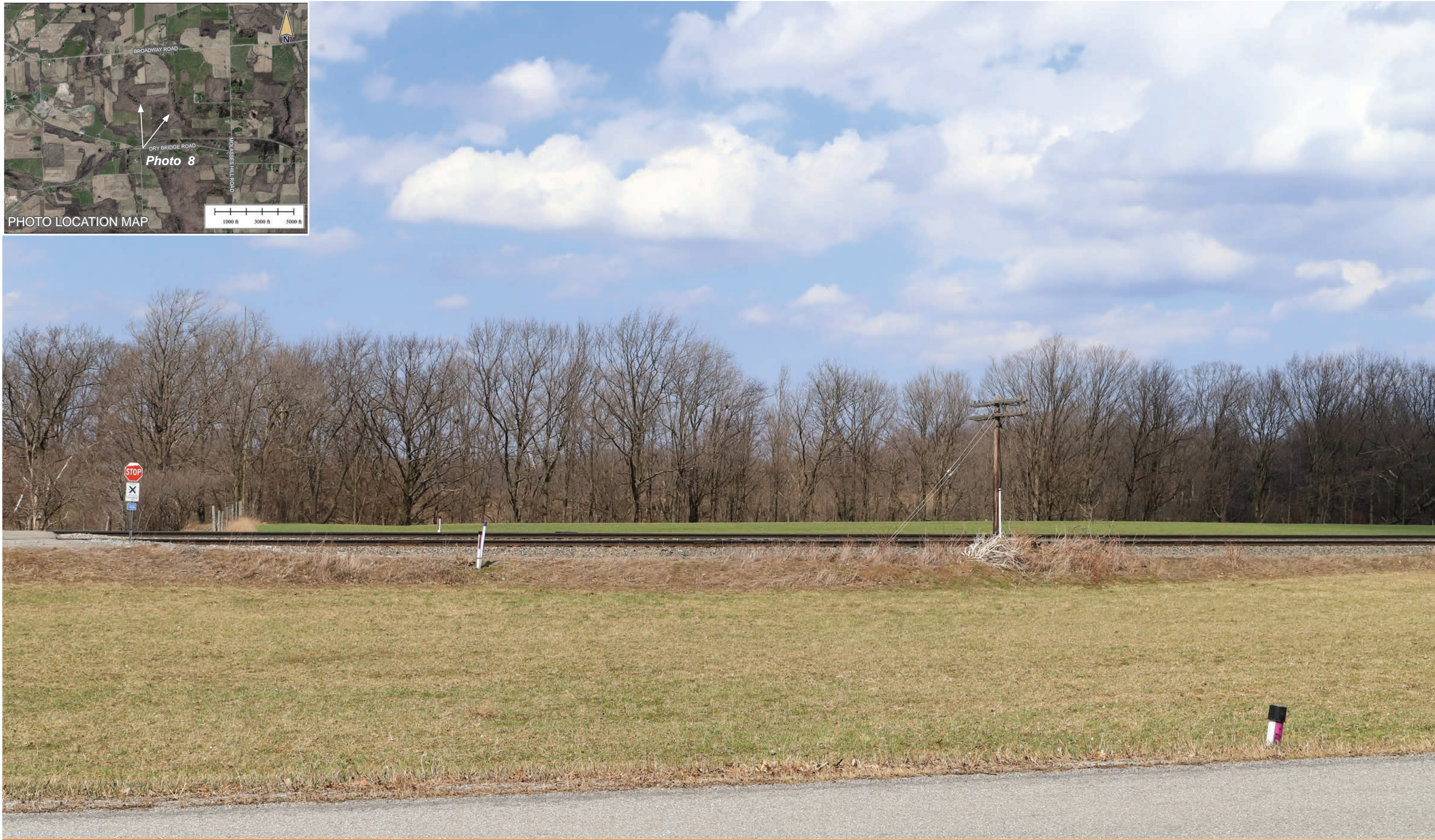
Photo 8 50mm - Dry Bridge Rd near # 3959 EXISTING CONDITION
