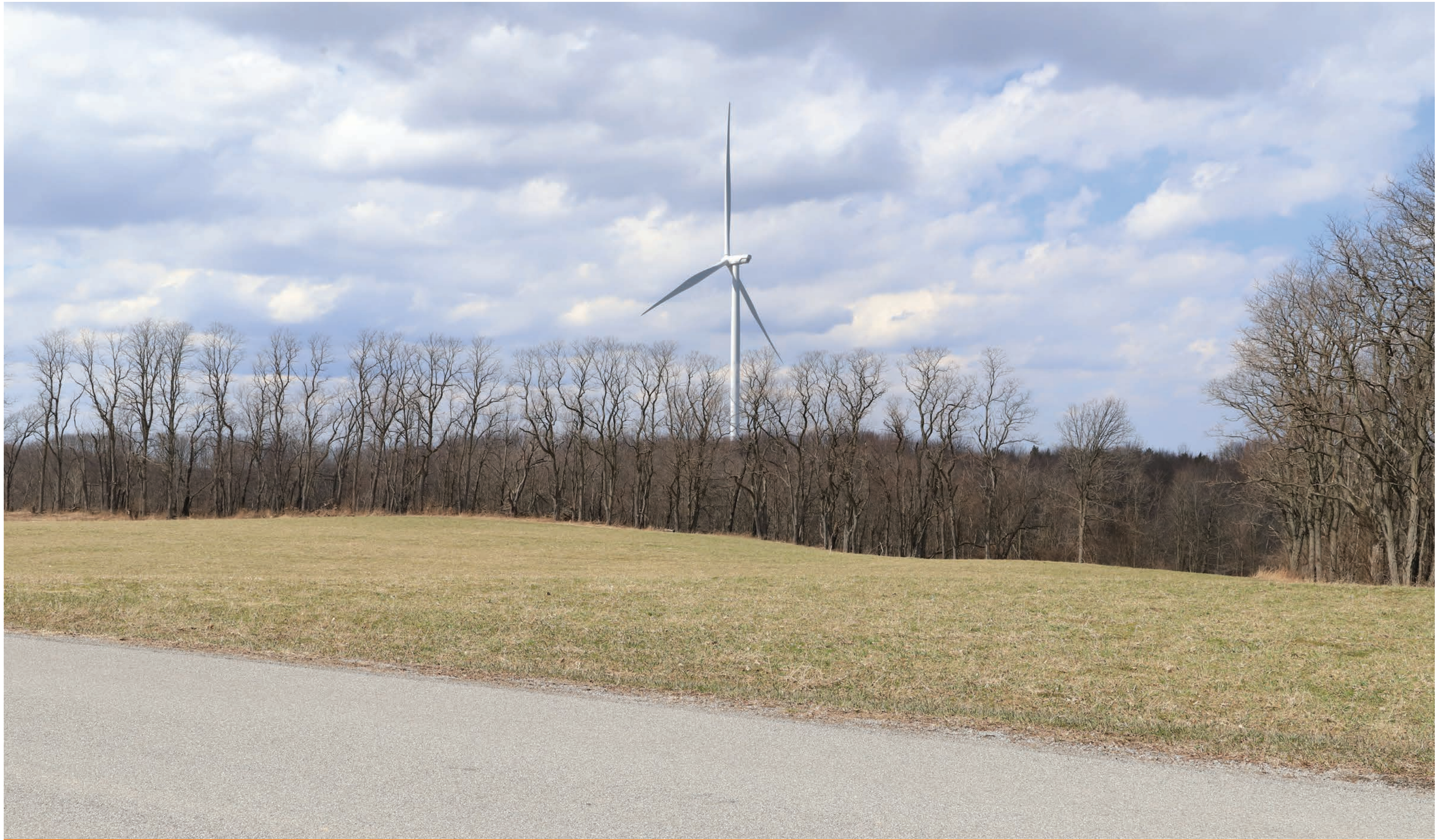
Photo 7 35mm - Dry Bridge Rd near # 4030 SIMULATED CONDITION - 640
