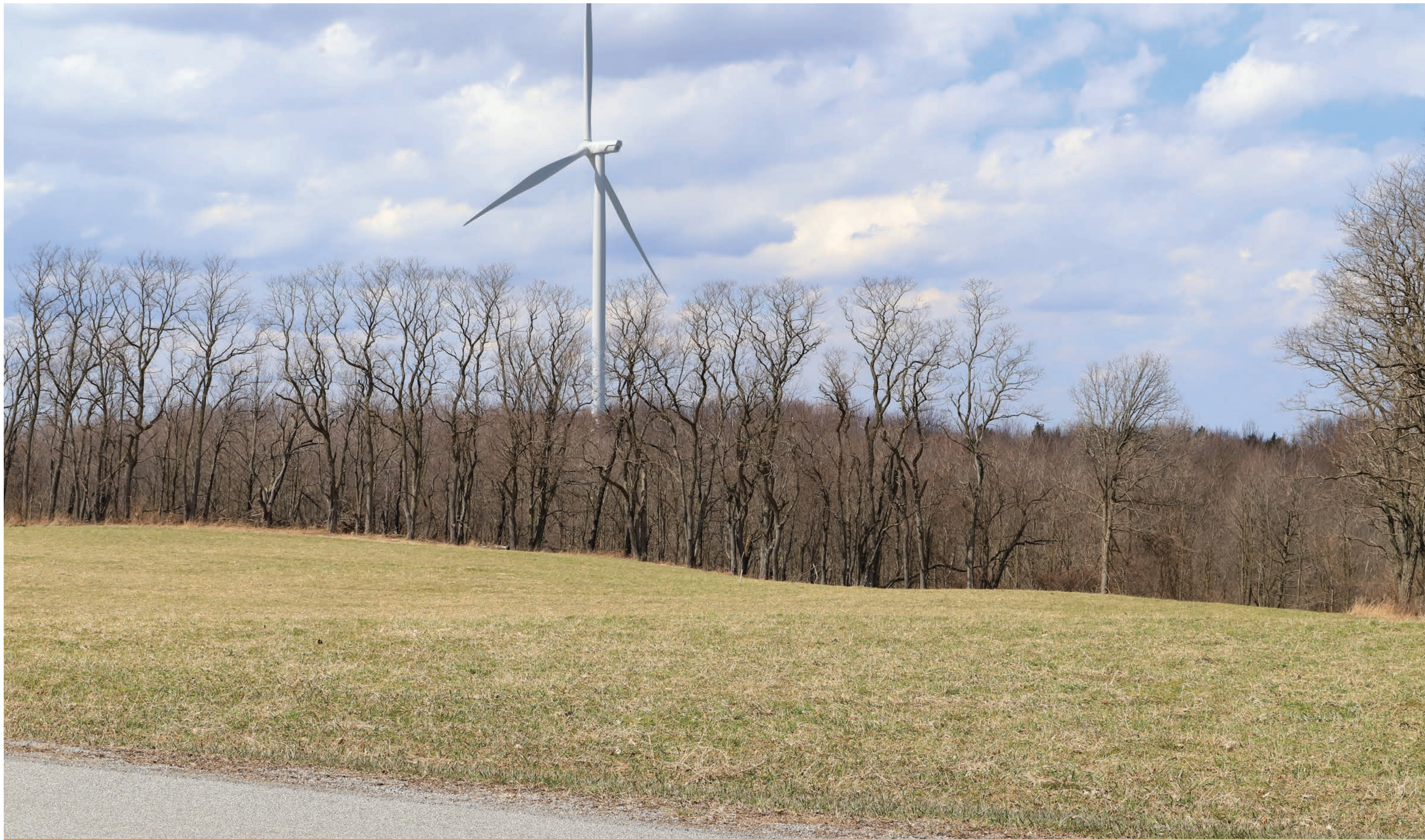
Photo 7 50mm - Dry Bridge Rd near # 4030 SIMULATED CONDITION - 640
