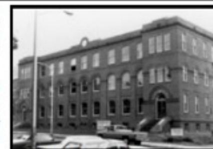
The school after rehabilitation. Windows, doors, and transoms were repaired. The building was not cleaned.
