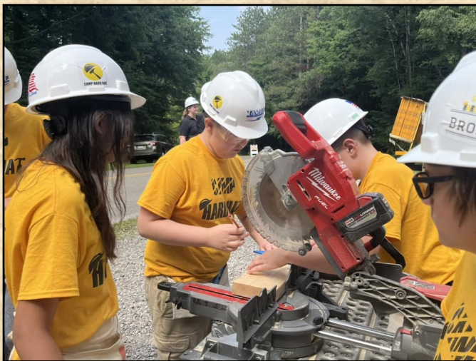
Campers measure and cut lumber
